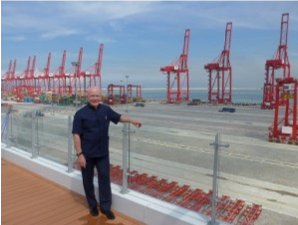
Chinese-built container terminal in Sri Lanka
