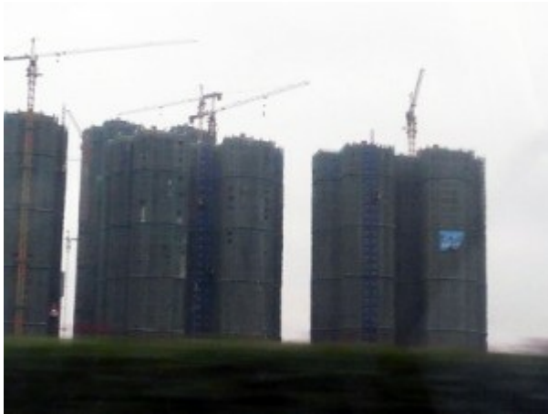
Construction in Wuhan, China
