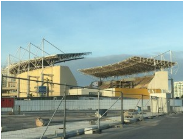
Olympic stadium under construction
